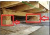
Place wooden supports under the pallet as the pallet is pulled out.
